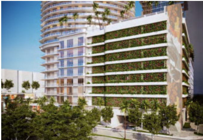
Current Flow Tower Ground View
